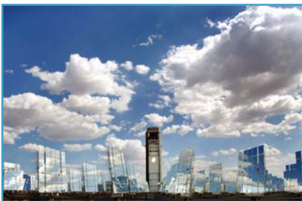
National Solar Thermal Test Facility at Sandia National Laboratories provides experimental engineering data for the design, construction, and operation of unique components and systems in proposed solar thermal electrical plants planned for large-scale power generation.
