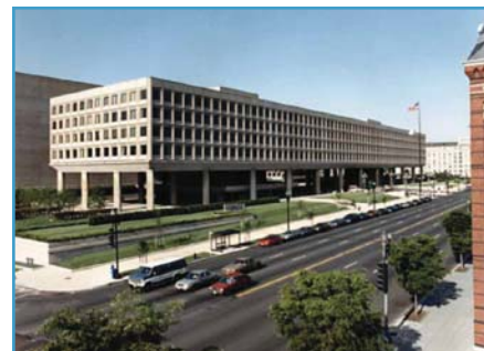
DOE Headquarters Forrester Building in Washington, D.C.
