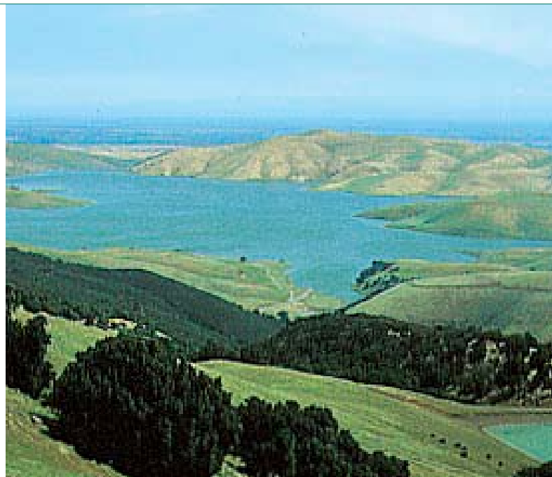
The Los Vaqueros Reservoir improves water quality and provides an emergency supply of water for all water providers listed in this report.
