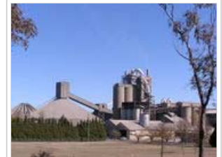
Blue Circle Southern Cement works near Berrima, New South Wales, Australia.
