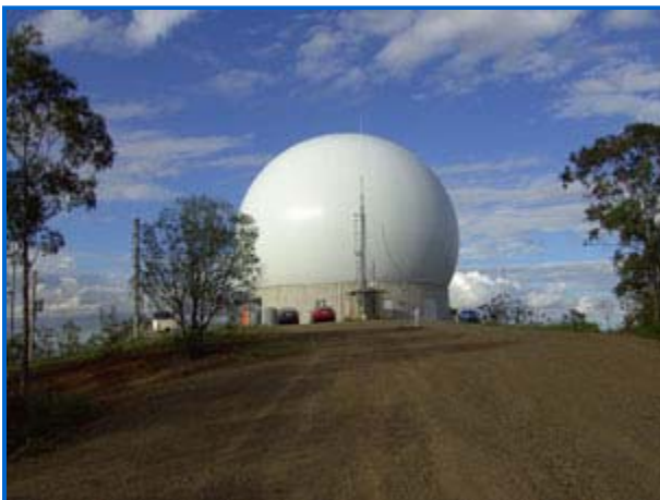
Figure 4: Photo of the CP2 radar at the Redbank Plains site. (click to enlarge)
