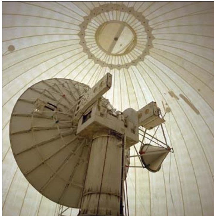
View inside the CP-2 radome near Fort Morgan. (Photo by Ginger Hein.)
