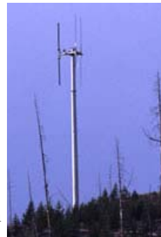
The illegal 100-foot cell phone tower overlooks Old Faithful in Yellowstone National Park.
