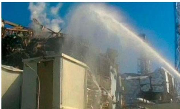
A fire truck sprays water at reactor 3 of the Fukushima nuclear power plant to help cool reactors and stop the spread of radiation. Photograph: Reuters
