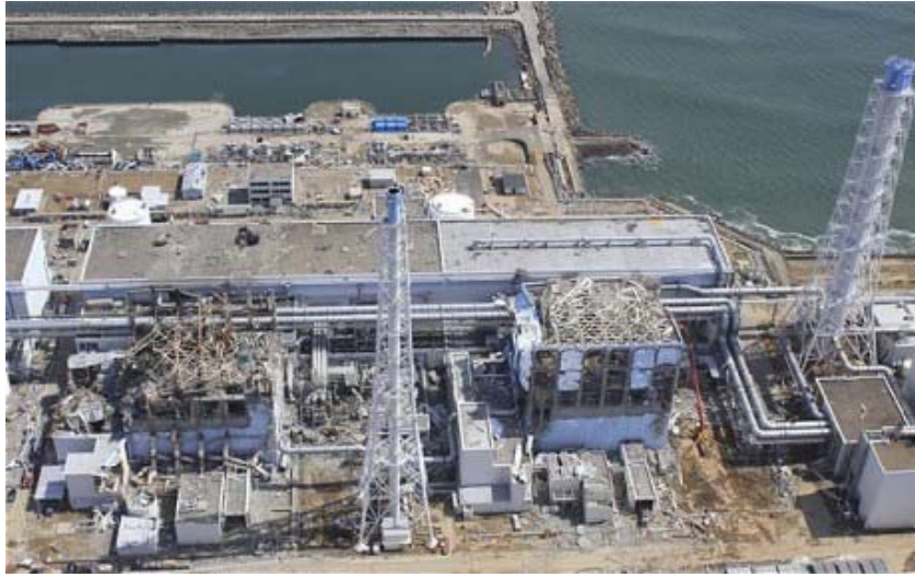
The damaged Unit 3 (left) and Unit 4 Photo: AIR PHOTO SERVICE/AP
