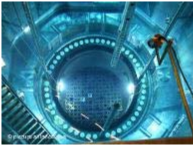
The reactor at Philippsburg
