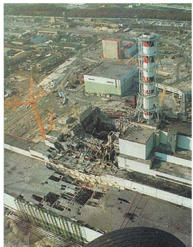
The nuclear reactor after the disaster. Reactor 4 (center). Turbine building (lower left). Reactor 3 (center right).
