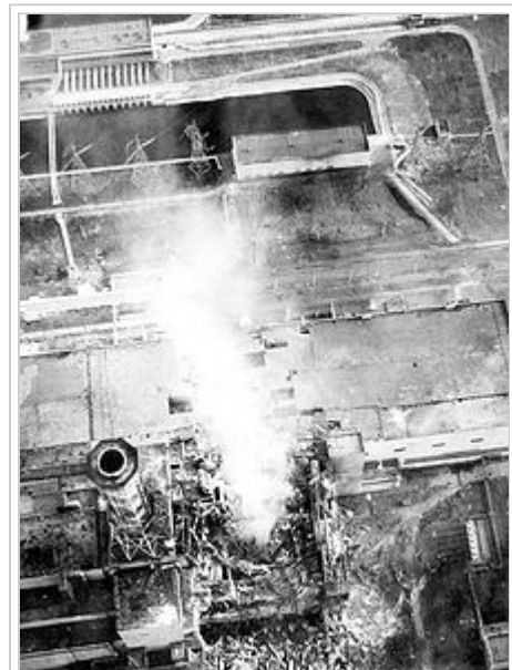
Aerial view of the damaged core. Roof of the turbine hall is damaged (image center). Roof of the adjacent reactor 3 (image lower left) shows minor fire damage.
