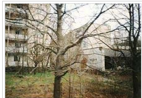
Abandoned housing blocks in Prip'yat
