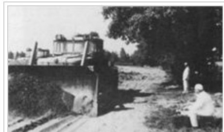
Radio-operated bulldozers being tested prior to use
