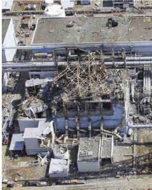
Figure 2: Reactor No. 3 Spent Fuel Pool Area
