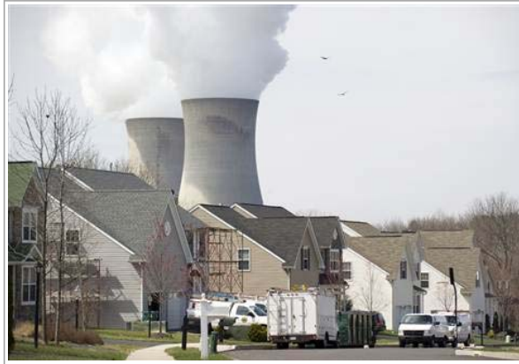
Stan Honda / AFP/Getty Images Cooling towers from the Limerick Generating Station, a nuclear power plant, 28 miles from Philadelphia, are seen from an nearby neighborhood. The population within 10 miles of the plant grew by 18.7 percent in the past decade.
