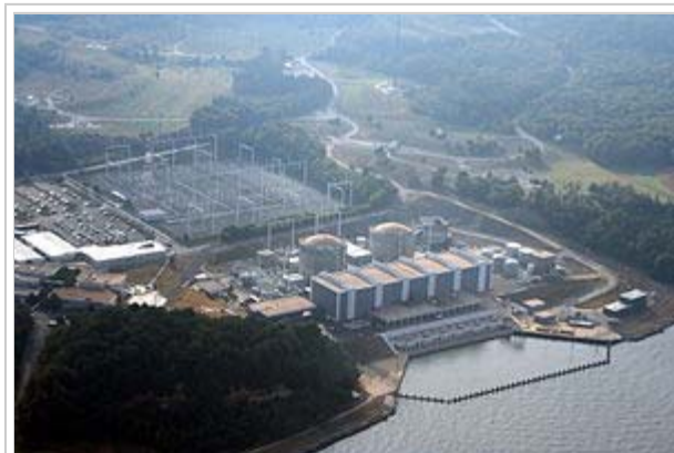
Calvert Cliffs Nuclear Power Plant
