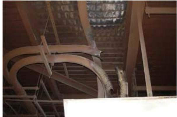
*Conduit for electrical cables damaged by the fire at the H.B. Robinson plant. (Photo courtesy of NRC)*
