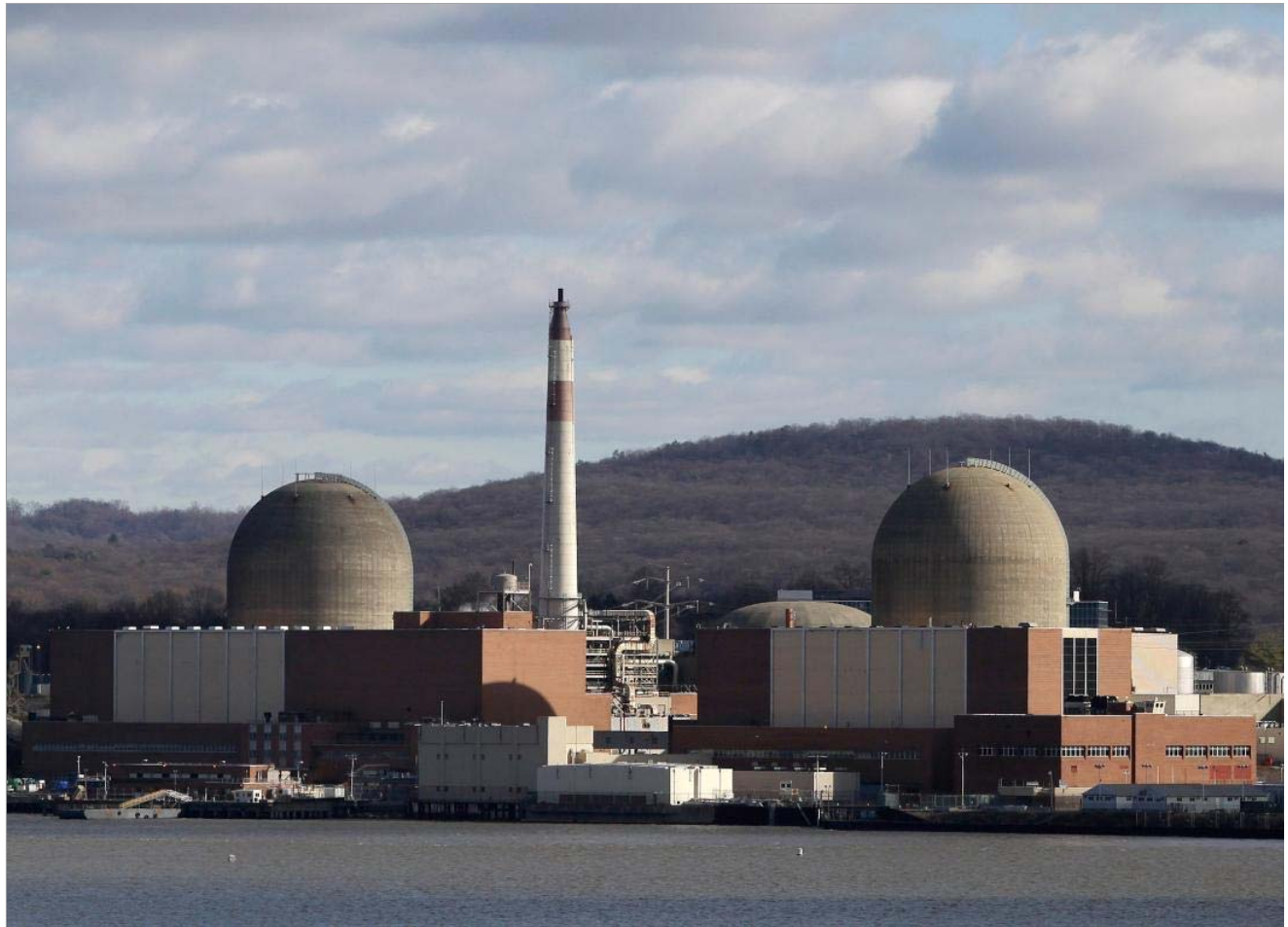
This Wednesday, Dec. 16, 2009 picture shows the Indian Point nuclear power plant along the banks of the Hudson River in Buchanan, N.Y., about 25 miles north of New York City. As of 2009, the smaller dome at center; the 36-year-old reactor 2 is at left and the 34-year-old reactor 3 is at right. Applications to extend the lives of pressurized water units 2 and 3 are under review by the Nuclear Regulatory Commission (NRC) (AP Photo/Jacobson)
