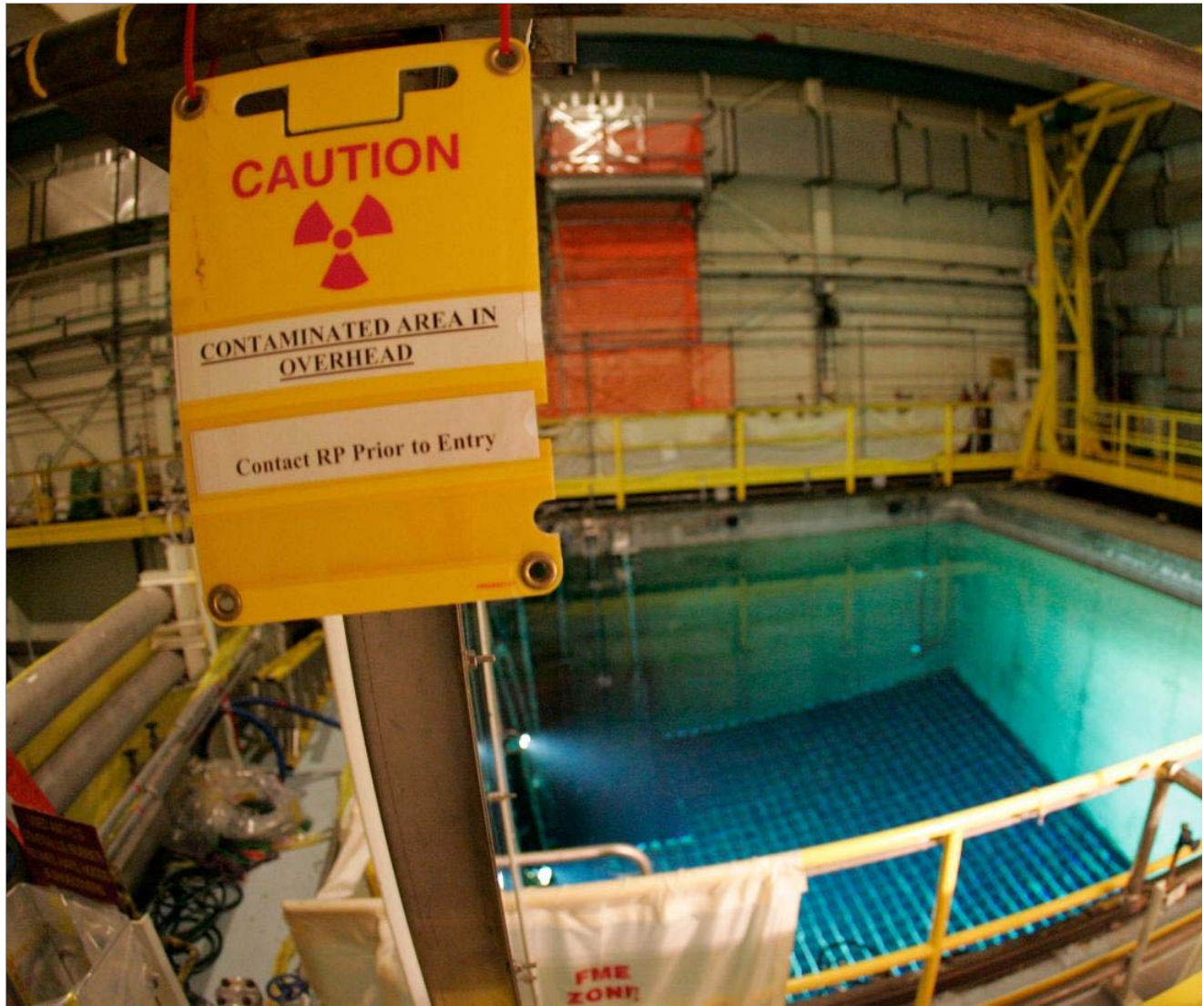
In this Friday, April 20, 2007 picture, a caution sign marks an area surrounding a pool that protects spent nuclear fuel at the Indian Point nuclear power station in Buchanan, N.Y. Because it failed to find a location for permanent storage of spent fuel, many tons of highly radioactive used reactor rods are kept in pools inside reactor containment buildings. (AP Photo/Julie Jacobs)
