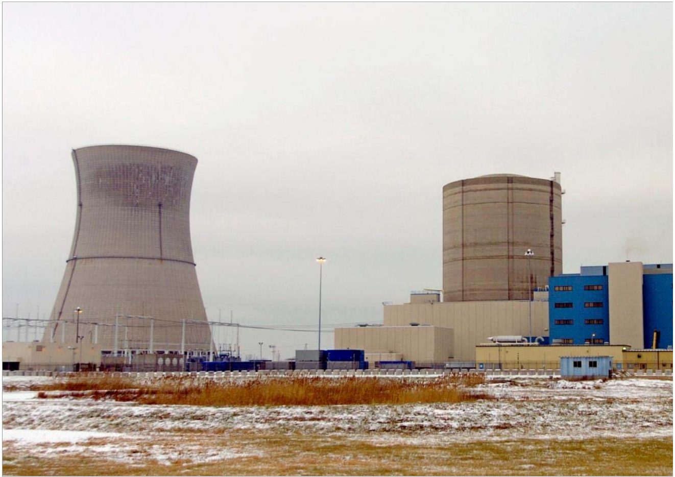
FILE - This Monday, Dec. 15, 2003 file picture shows the then-idled Davis-Besse nuclear power station in Oak Harbor, Ohio. The Davis-Besse plant was shut down for two years starting in 2002 after workers found an acid leak that nearly ate through a steel cap on the reactor vessel at the plant. It was the most extensive corrosion seen at a U.S. nuclear reactor. (AP Photo/Mark Duncan)
