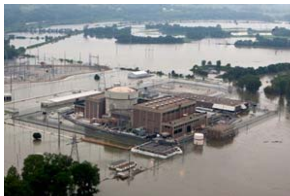
The Fort Calhoun nuclear power station, in Fort Calhoun, Neb., is surrounded by flood waters from the Missouri River on June 14, 2011. (Nati Harnik/AP Photo)
