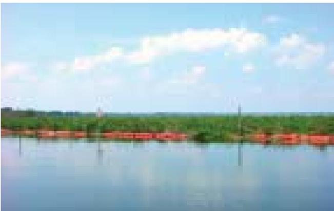
*Barrier constructed across Lake Hancock outfall canal to prevent floating islands from clogging flood control structure*
