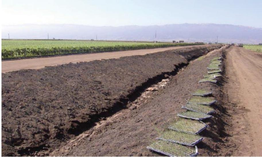
**Figure 3. Graded ditch, with trays of grass plugs.**
